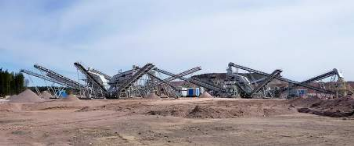
PITKYARANTA (Russia) – Granite/amphibolite processing plant 500 tph
